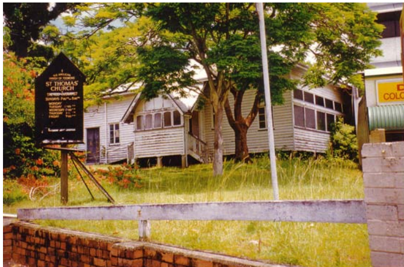
St Thomas' Church Hall – 67 High Street, Toowong
