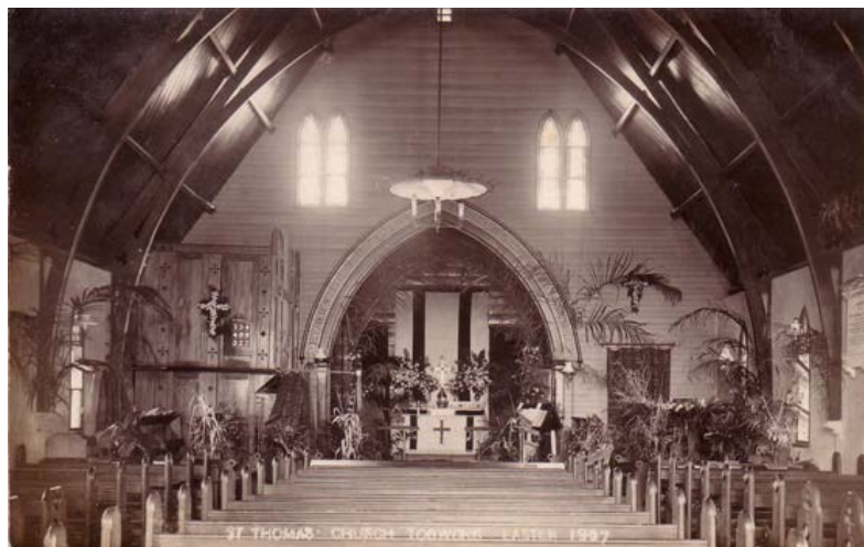
Interior of the old wooden Sanctuary
