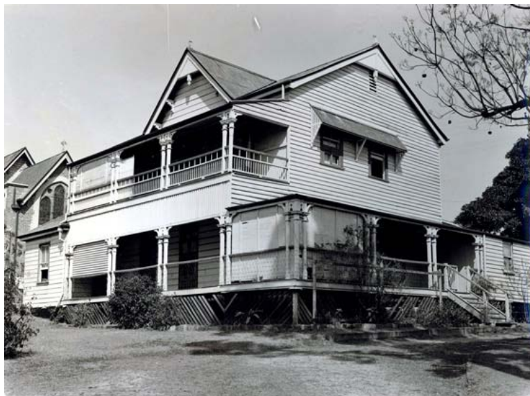
The first St Thomas' Rectory showing the second storey added at the turn of the century.
